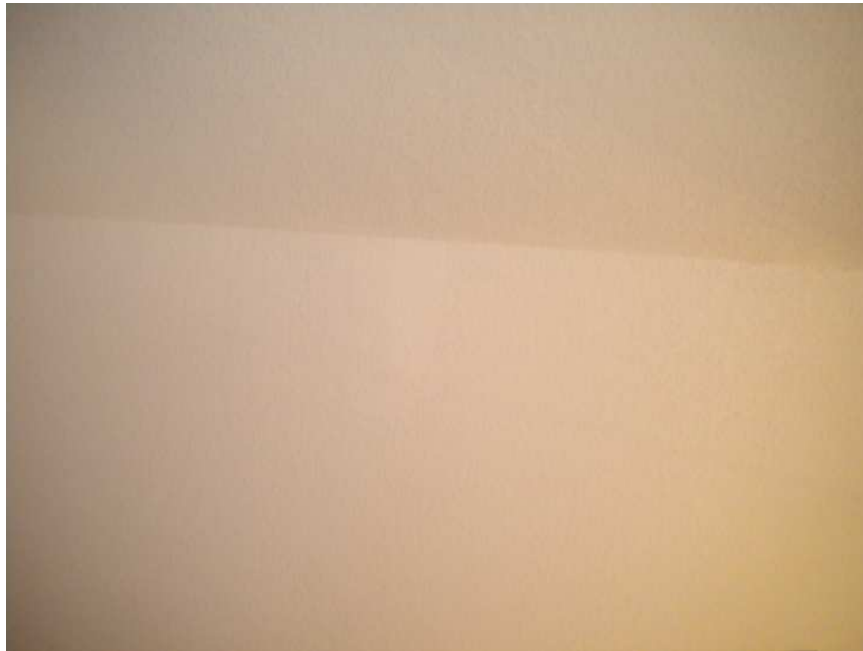
View of Ceiling@ Kitchen/Dining
